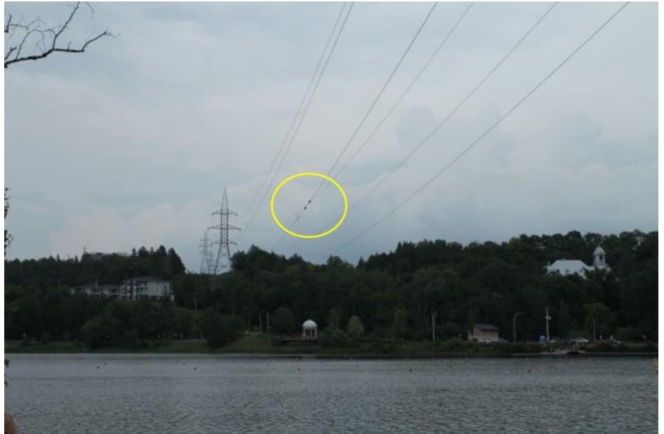
Figure 2: Photo of the damage to the lower cable of the power line (Source: TSB)
