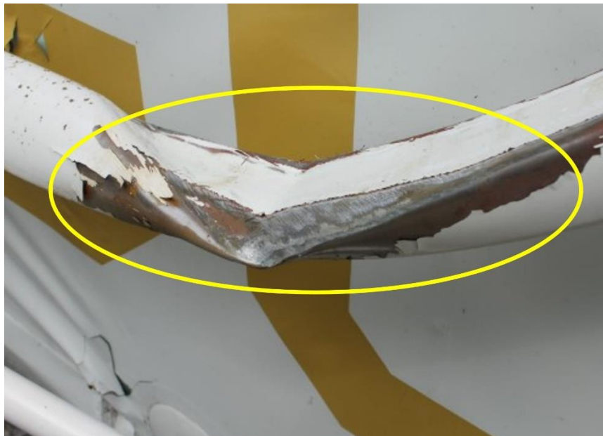
Figure 4: Photo of the damage to the left-wing strut caused by the collision with the cable (Source: TSB)
