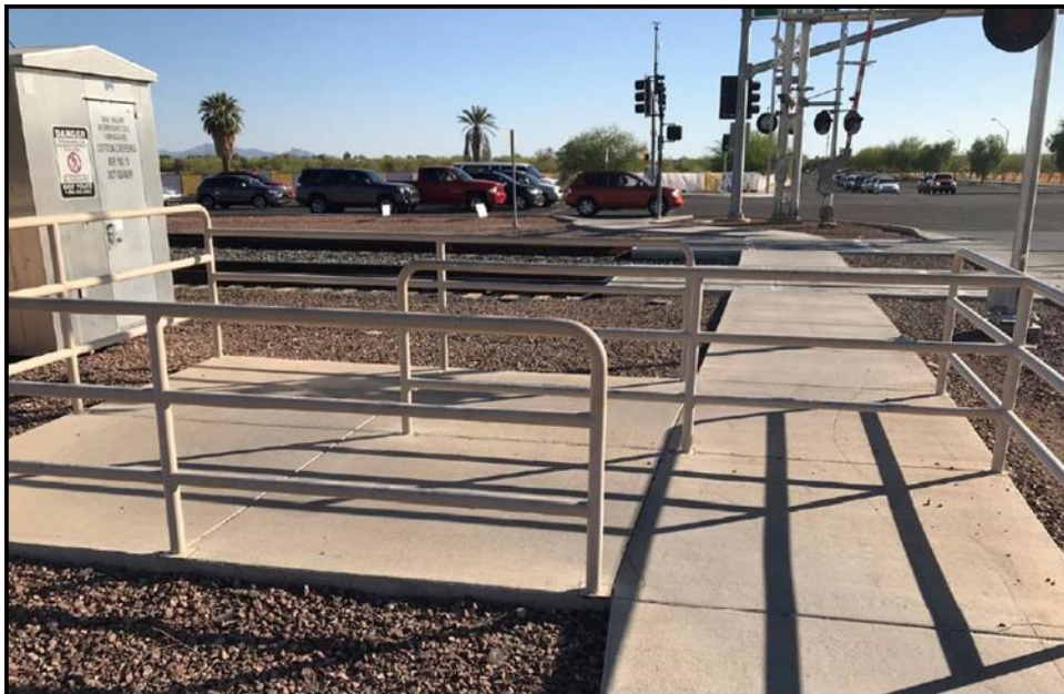
Figure 26-2 Example image of Pedestrian Maze Barrier for Public Grade Crossing
