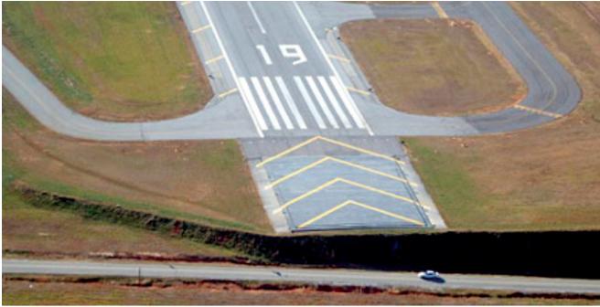
(The EMAS bed is the grey area under the yellow chevrons)
