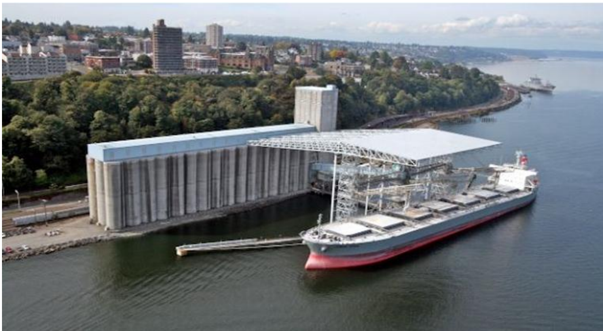
Exhibit 2: Permanent Roof Structure at Export Terminal
