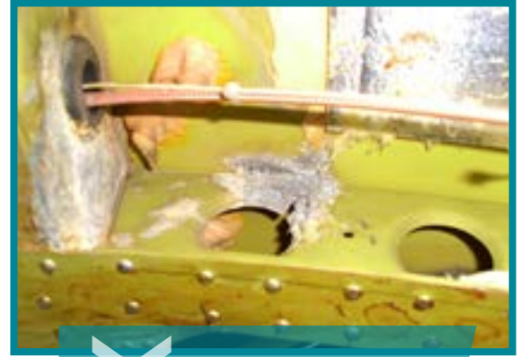
Severe Surface Corrosion Discovered on the Fuselage Lower Longeron
