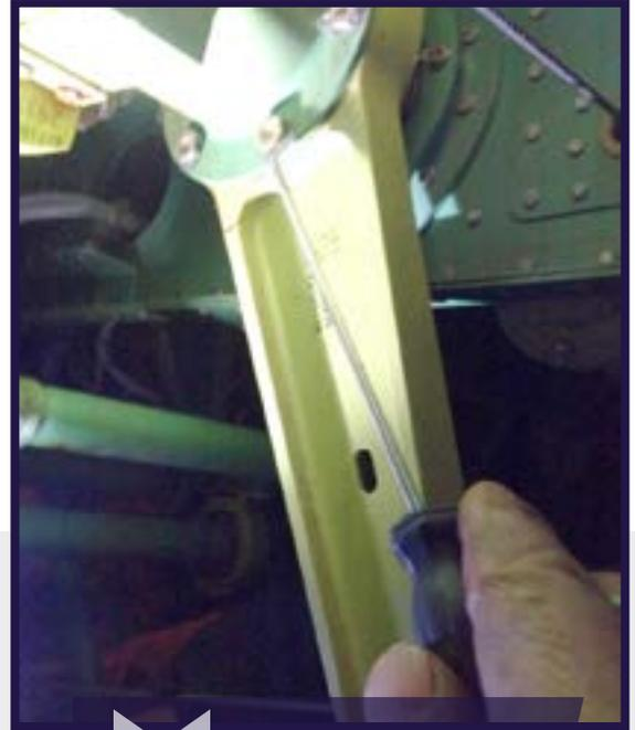
Improperly torqued hardware allowing nuts to be left loose
