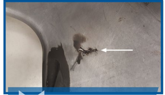
Damage on the spinner caused by the propeller de-ice wires.
