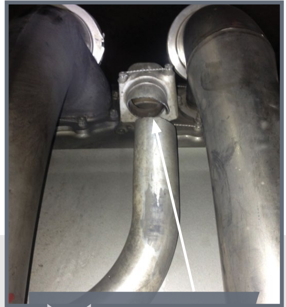
Missing engine cowl blow-out panel and failed anti-ice duct
