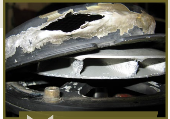
Alternating current generator internal impeller and backshell damaged from a nut
