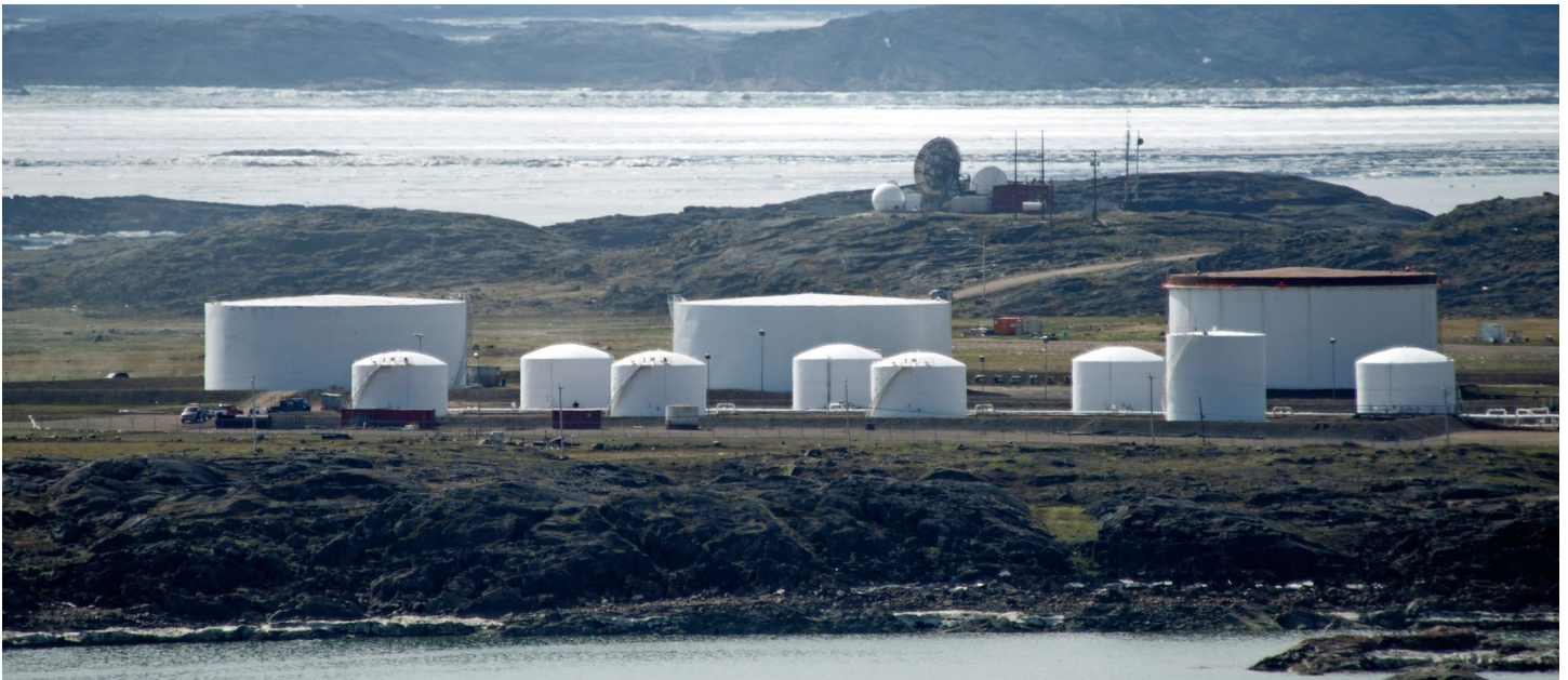
Oil handling facility in Iqaluit, Nunavut.
